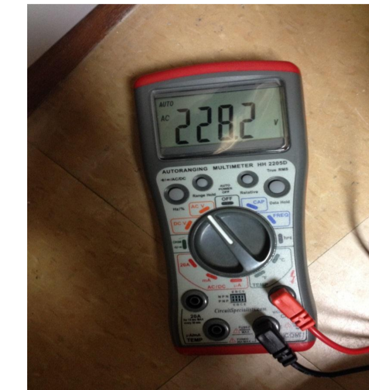
Outlet voltage is 228.8 V.
